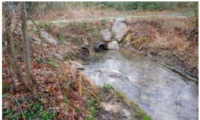
Culverts PAN & Stream Partners Provided
